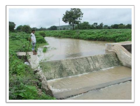
This check dam helps detain stream water for longer periods and increase recharge of ground water.
